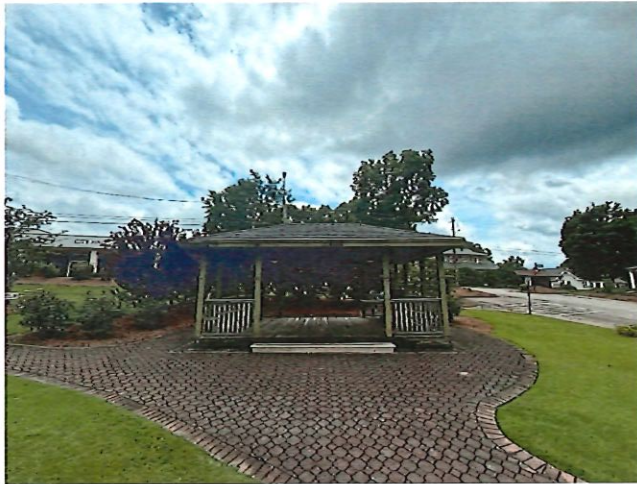
Existing Structure Referenced.
